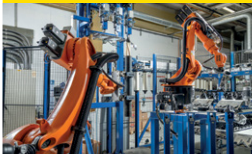
Automatic operation management of robots and AGVs
